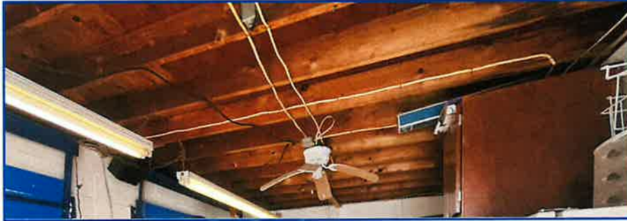
No evidence of water damage to roof/ceiling structure
