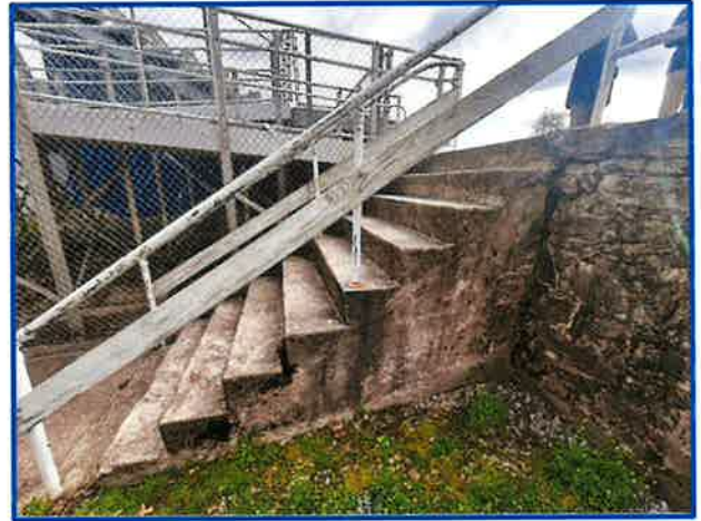
Stairs help to stabilize wall movement
